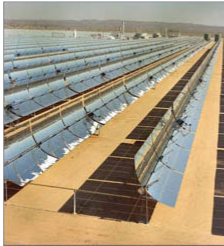
Figure 2: Parabolic trough system.
