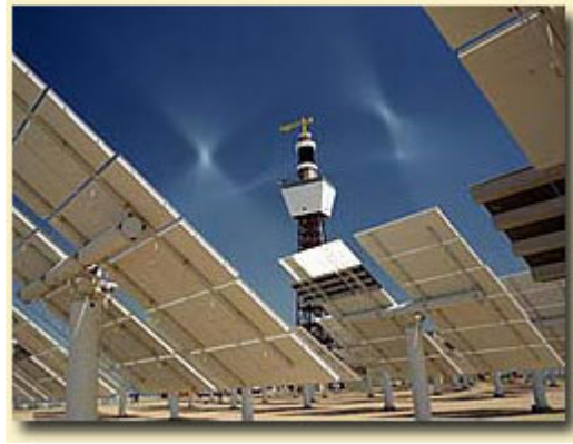
Figure 4: Power tower system
