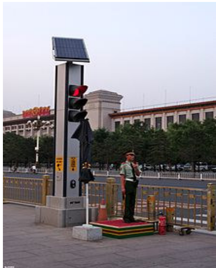
Solar powered Traffic signal
